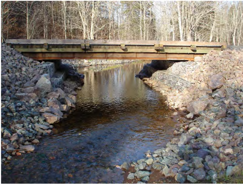
New bridge installation, Paul MacDonald, PHP
